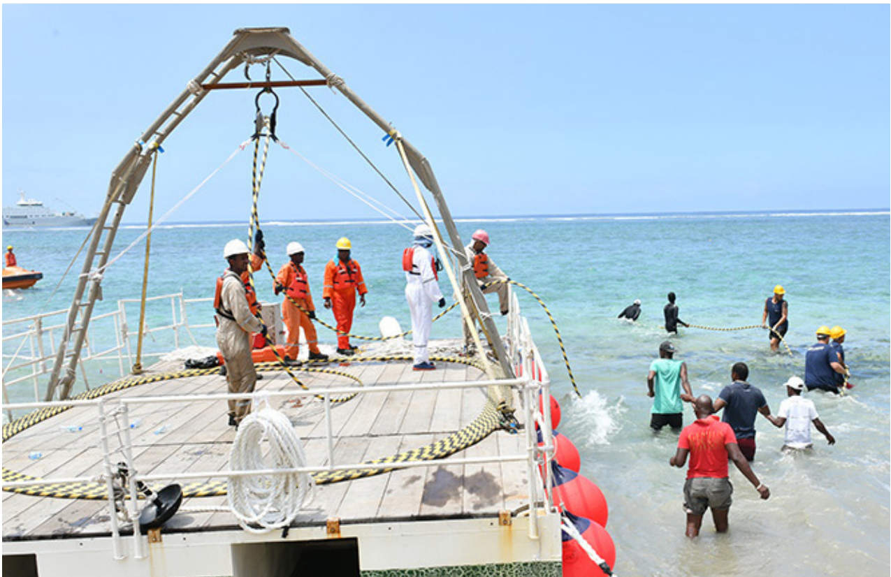
Installing MARS cable in Rodrigues
