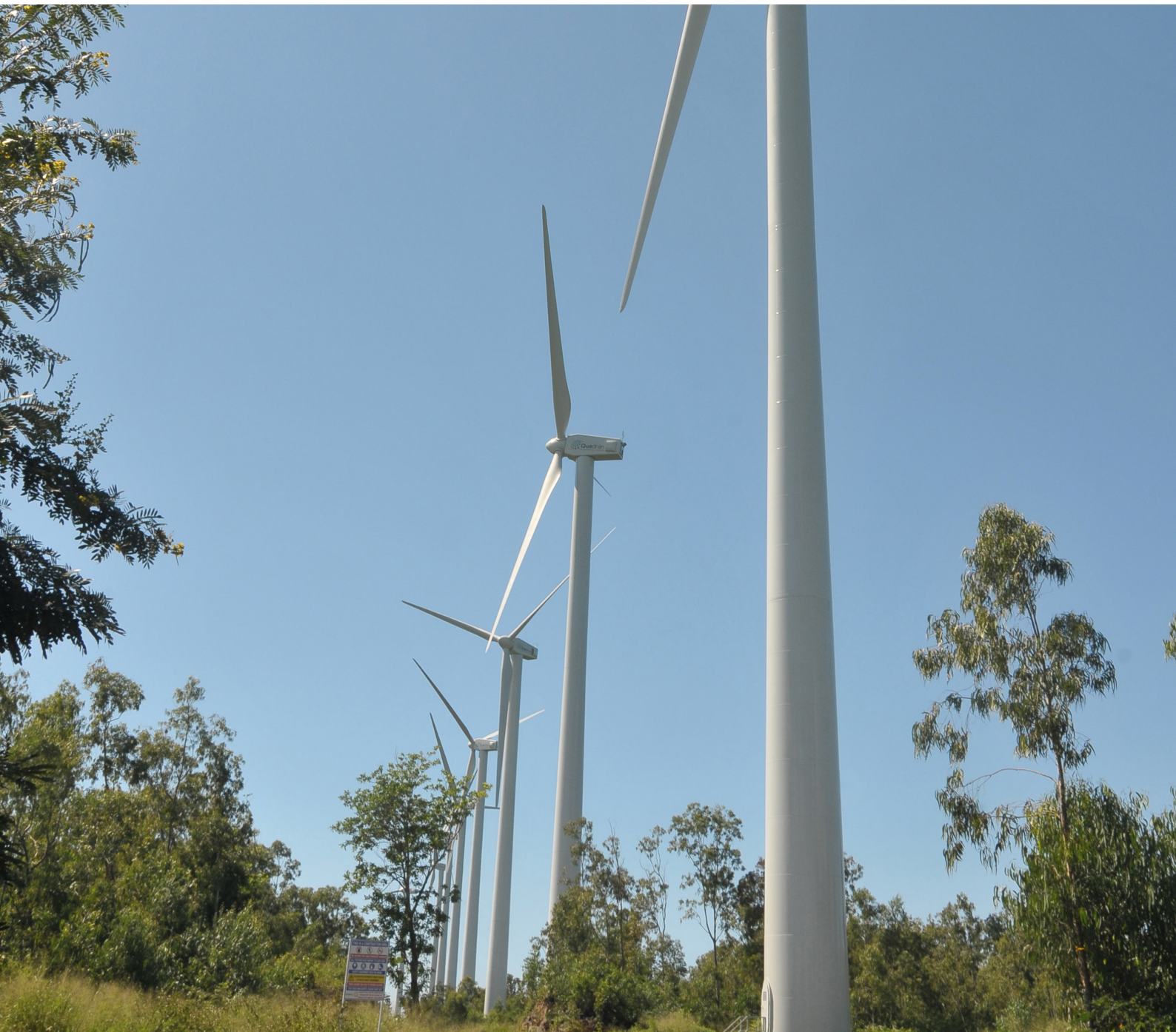
Wind Farm at Plaine des Roches
