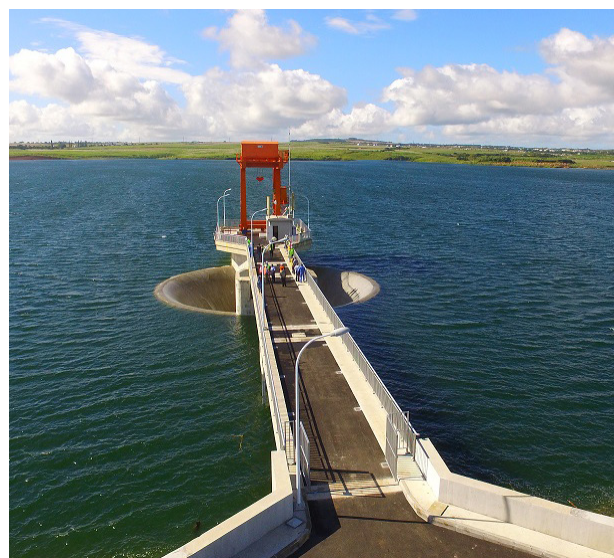
New Bagatelle Dam constructed in 2017
