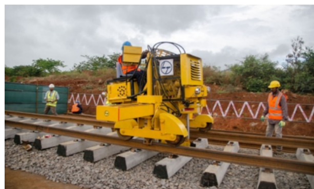
Metro Express Works in Mauritius
